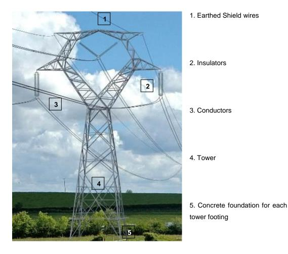
Figure 6.25: General Arrangement of a C-IVI-1 (IVI) Tower
